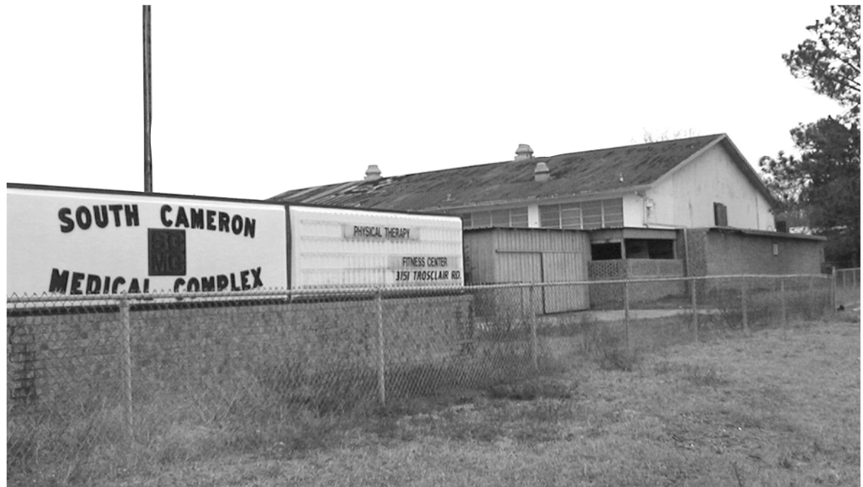
THE CAMERON PARISH School Board is offering to lease the old Audrey Memorial School on Trosclair (Front Ridge) Road. After the closing of the school the building was later used for a trade school and several years ago was a physical therapy facility for the South Cameron hospital.
