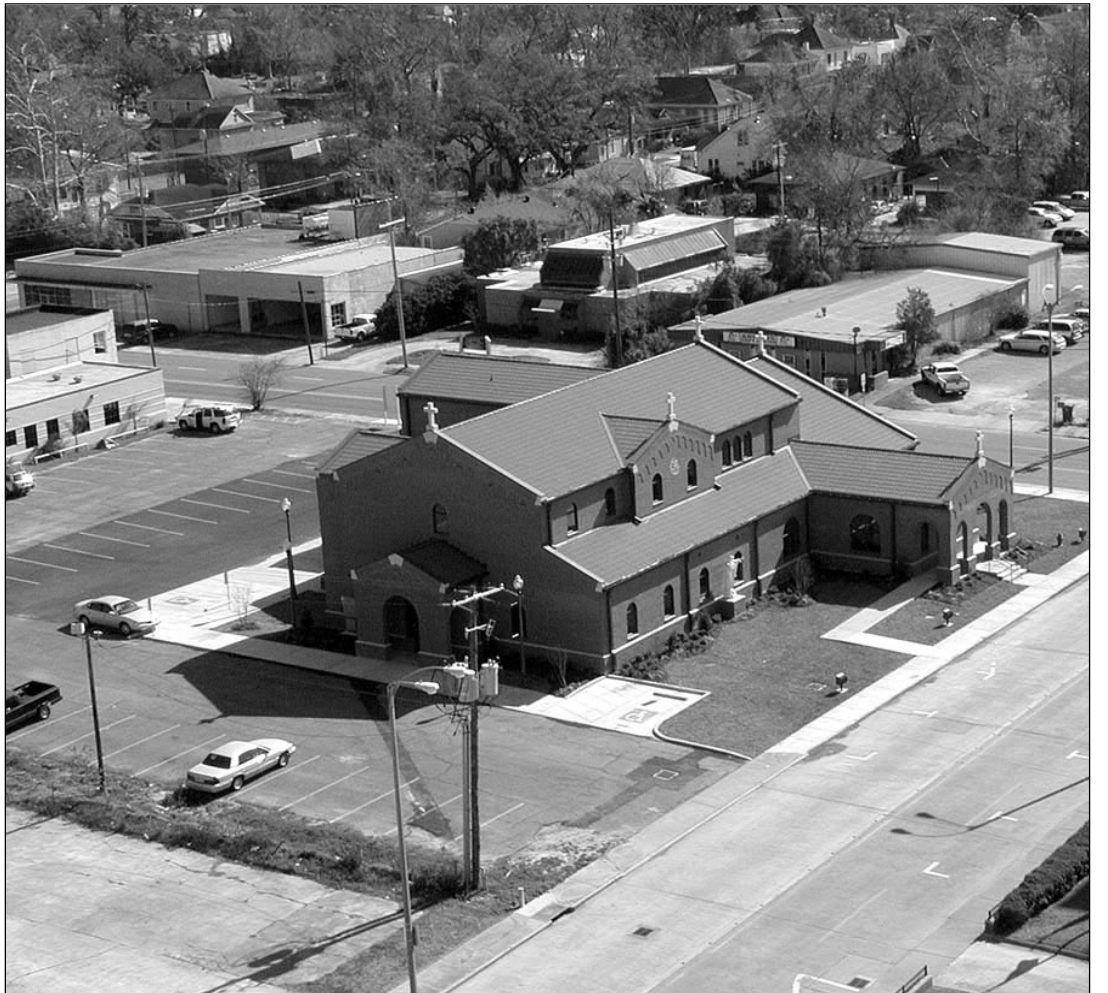
A birds eye view of the newly completed office building for the Cathedral of the Immaculate Conception in downtown Lake Charles from the top of City Hall shows the architecture of the building emulates the Lombardy-Romanesque style of the Cathedral. Dedication ceremonies are set for Feb. 19, following the 11:15 a.m. Mass. Open houses will be held on the weekend of Feb. 25-26 following each day's masses.
