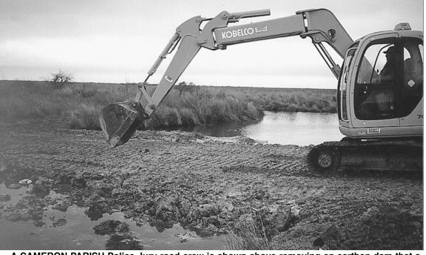
A CAMERON PARISH Police Jury road crew is shown above removing an earthen dam that a landowner had placed across a roadside ditch at Rutherford Beach. A Police Jury permit and the installation of a culvert are required for such work. (Photo by Geneva Griffith.)
