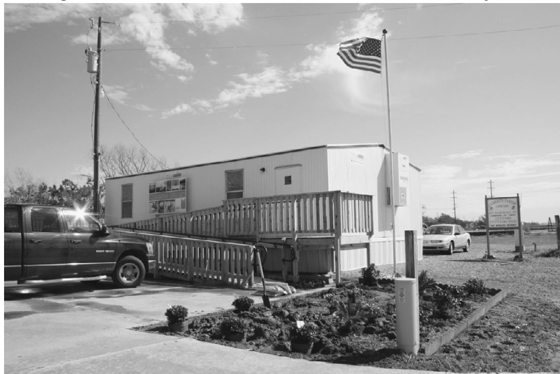
LANDSCAPING IS being installed at the Cameron Library in preparation for the Grand Opening on Monday. (Photo by Cyndi Sellers.)
