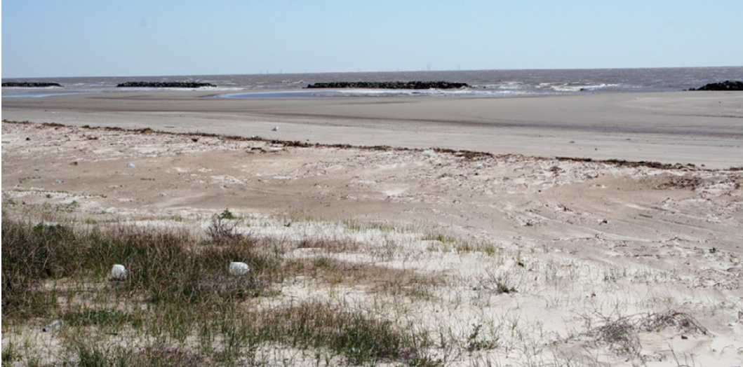
EXTREME LOW TIDE on Tuesday shows the tons of sand that have built up behind the newest set of breakwaters near Holly Beach. (Photo by Cyndi Sellers.)
