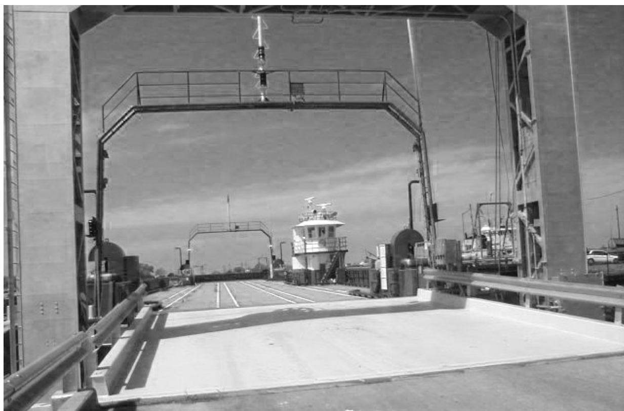
THE 50-CAR Cameron Ship Channel ferry is back from dry dock where it has been undergoing repairs for the past eight months. It will go back into operation as soon as a Coast Guard inspection is completed. A smaller, side-loading ferry has been in use in its place.
