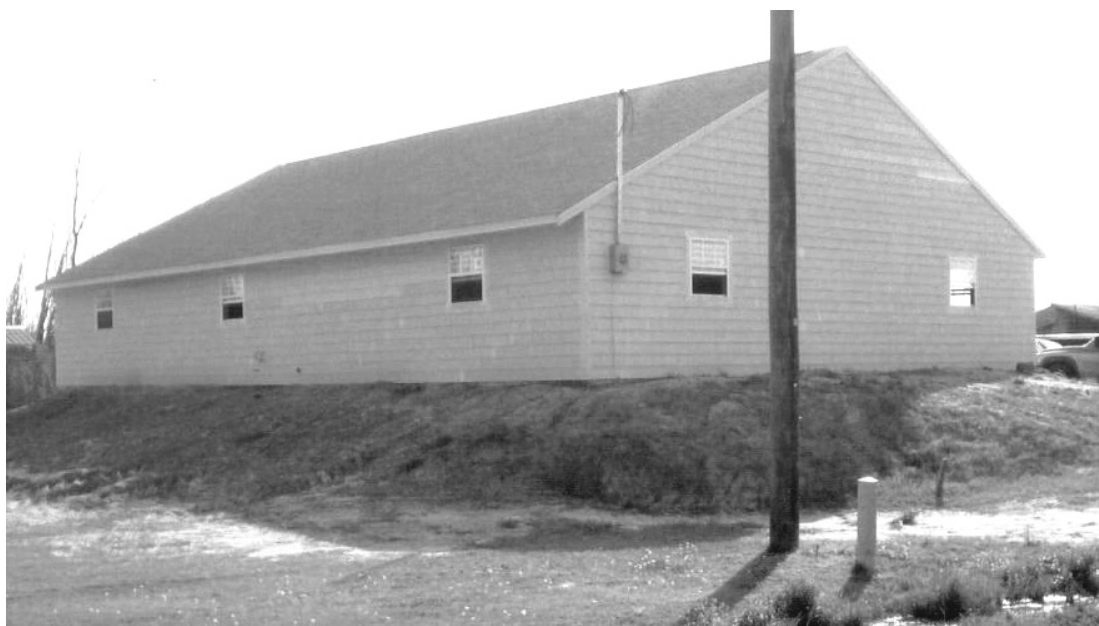
THE UNITED METHODIST Church members have been in the Hackberry area helping residents rebuild. Ronnie and Teresa (Pebbles) Nunez and their family have a new home that was built through this effort. The church members started the construction on February 24 and by March 10 all the outside was complete. The group will be working this week on the inside to try to complete the residence. Dalton Nunez, son of Ronnie and Pebbles, gave a grand tour of the residence.
