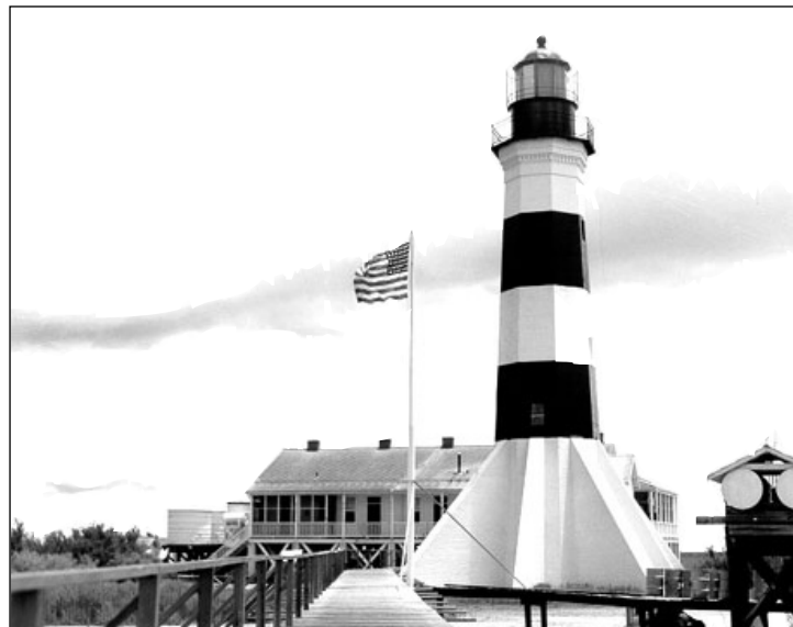
THIS PHOTO of the Sabine Pass Lighthouse in western Cameron Parish was taken years ago. The lighthouse keeper's house, shown in the background, has since burned. The Cameron Preservation Society has been working for a number of years to restore the lighthouse and to open the site to the public.
