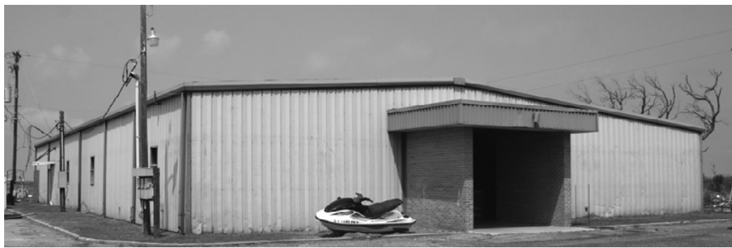
CAMERON MULTI-PURPOSE building, one of the least damaged public buildings after Hurricane Rita, is finally on track for repair, with plans currently being developed for renovation. (Photo by Cyndi Sellers.)
