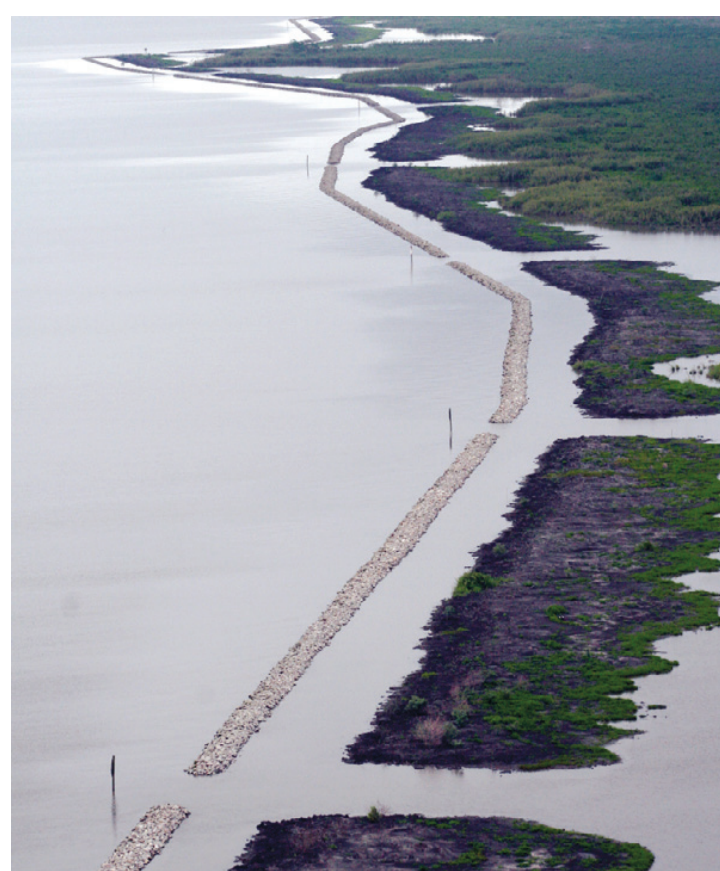
ROCK BARRIERS now protect the south shore of White Lake in Vermilion Parish as a result of a Coastal Wetlands Planning, Protection and Restoration Act (Breaux Bill) project. (Photo by Cyndi Sellers.)
