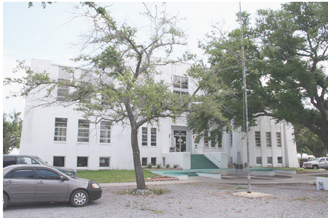
BUILT IN 1938 as a Public Works Administration project, the Cameron Parish Courthouse has withstood two devastating hurricanes in the past half century--Audrey in 1957 and Rita in 2005. This recent photo shows the fortress like strength of the building. The trees in the foreground were planted after Audrey. The building will be washed prior to the Audrey 50th anniversary on June 27. (Photo by Cyndi Sellers.)
