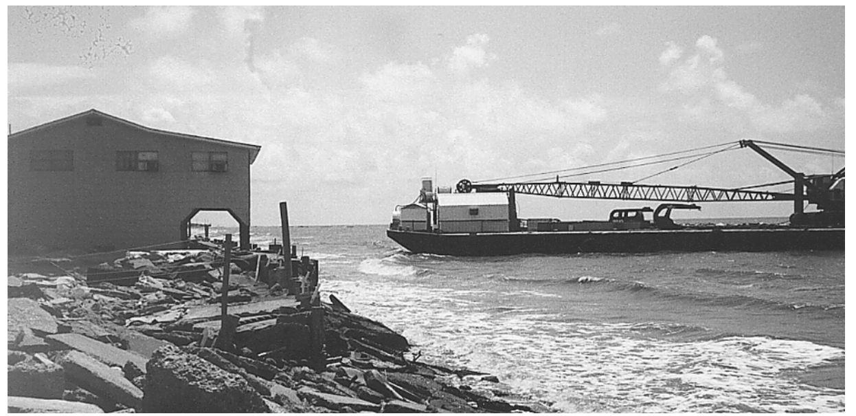
THIS LARGE BARGE and dragline has arrived at Constance Beach in preparation for a $20 million shore restoration project in the Holly-Beach-Constance Beach area. The breakwaters currently in place will be built up and sand will be pumped on to the beach. (Photo by Geneva Griffith.)
