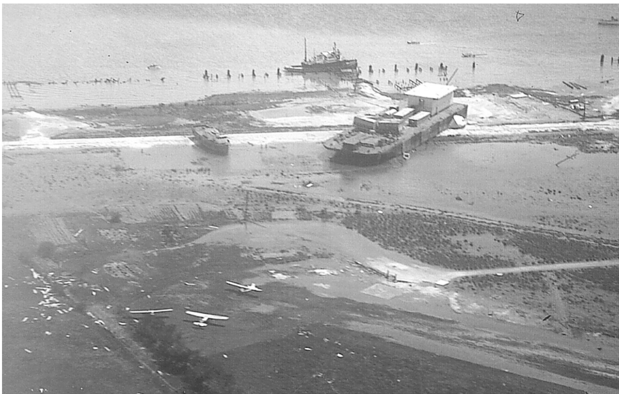
WEDNESDAY, June 27 will be the 44th anniversary of Hurricane Audrey which devastated Cameron Parish in 1957. The above photo, furnished the Pilot by Conway LeBleu, shows a boat and a barge that were washed up on the road at Cameron by the storm. In the foreground was the Cameron airstrip.
