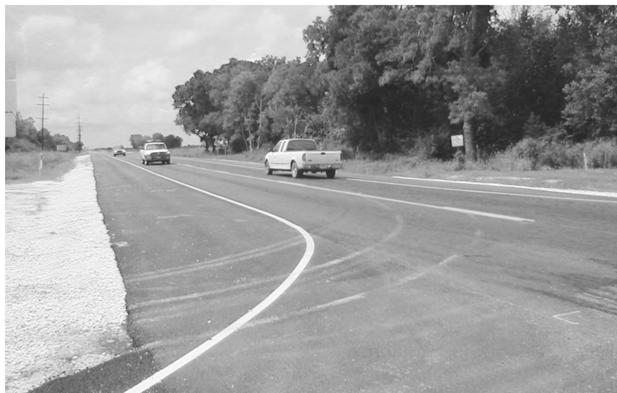
THE PROJECT to widen Hwy. 27 between Hackett's Corner and the Gibbstown Bridge has been completed and was dedicated last week. The expanded highway will provide for an additional lane of traffic to be used in the event of a hurricane evacuation from lower Cameron Parish.
