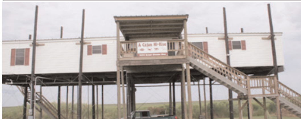
THIS MOBILE HOME, "Cajun High Rise" is located on the grand Chenier Highway and provides a good view of the elevation now required by FEMA regulations for trailers and homes in lower Cameron Parish. (Photo by Cyndi Sellers.)
