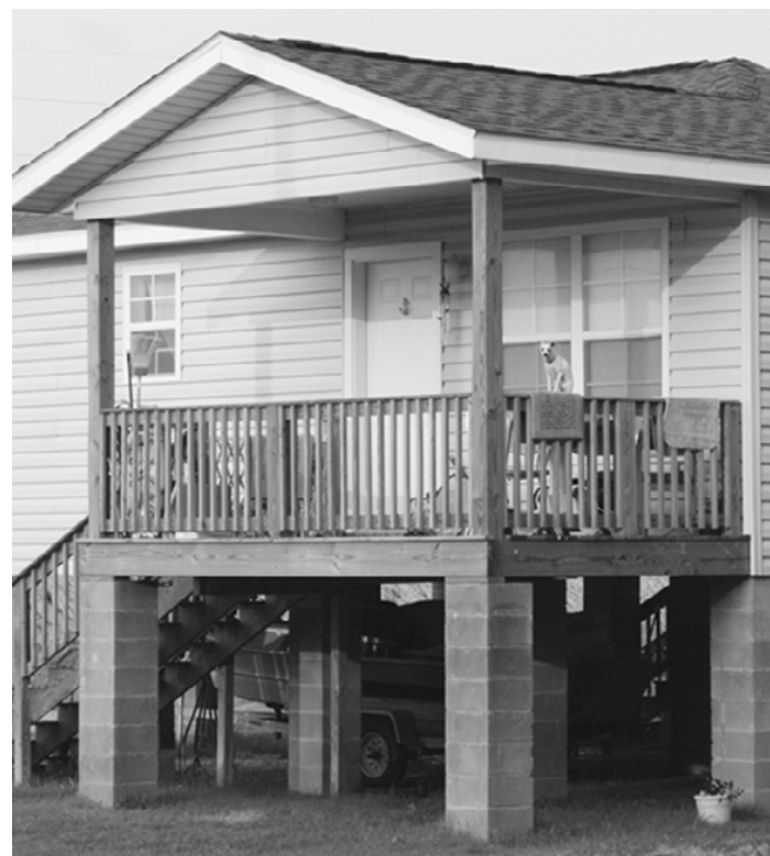
GUARDING THE Darlene Crosby home in Cameron is this small chihuahua. The home, like all other new ones, must be elevated to meet new building codes. (Photo by Cyndi Sellers.)
