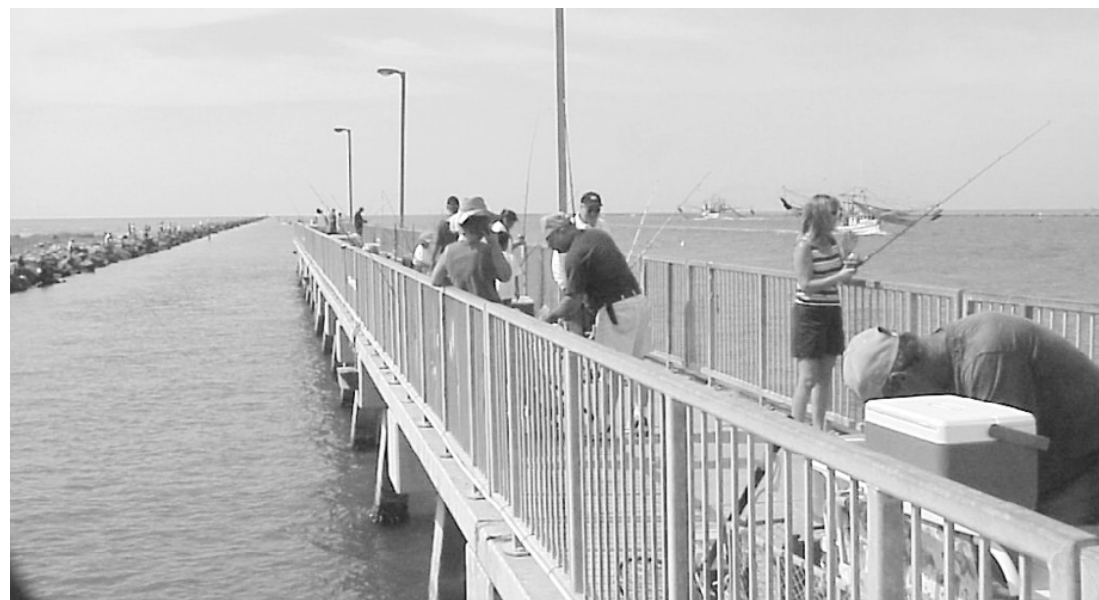
MUCH OF THE fishing in the Cameron Saltwater Fishing Rodeo this weekend will be from the Jetty Pier which was constructed several years ago along the east jetties on the ship channel. The pier offers a convenient place to get in some salt water fishing and large fish are caught regularly from the pier. (Photo by Cyndi Sellers.)
