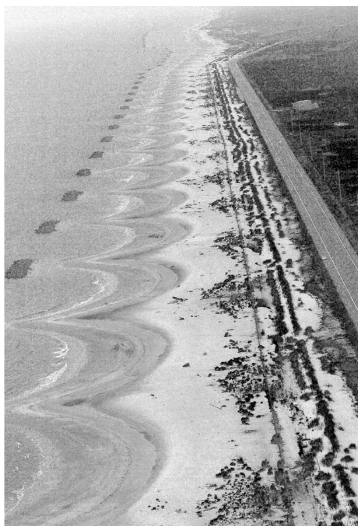
THIS PHOTO shows how the beach between Holly and Constance Beaches in Cameron Parish has built up since the stone breakwaters, on the left, were installed some years ago. White sand has also been pumped in on the beach from offshore. The Holly Beach-Johnson Bayou road can be seen on the right.
