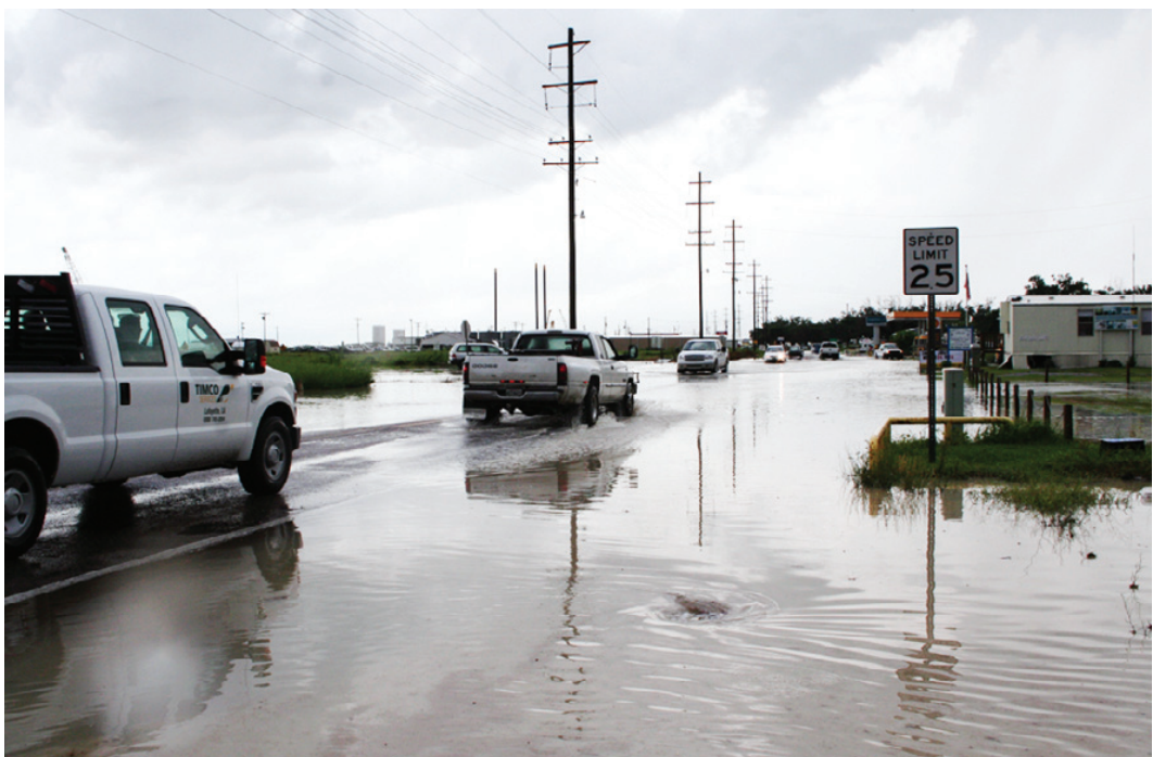
NO, IT'S NOT a tropical storm. This flooding on Cameron's main street last Thursday was caused by excessive rainfall as a line of thunderstorms trained over the town for nearly two hours. (Photo by Cyndi Sellers.)
