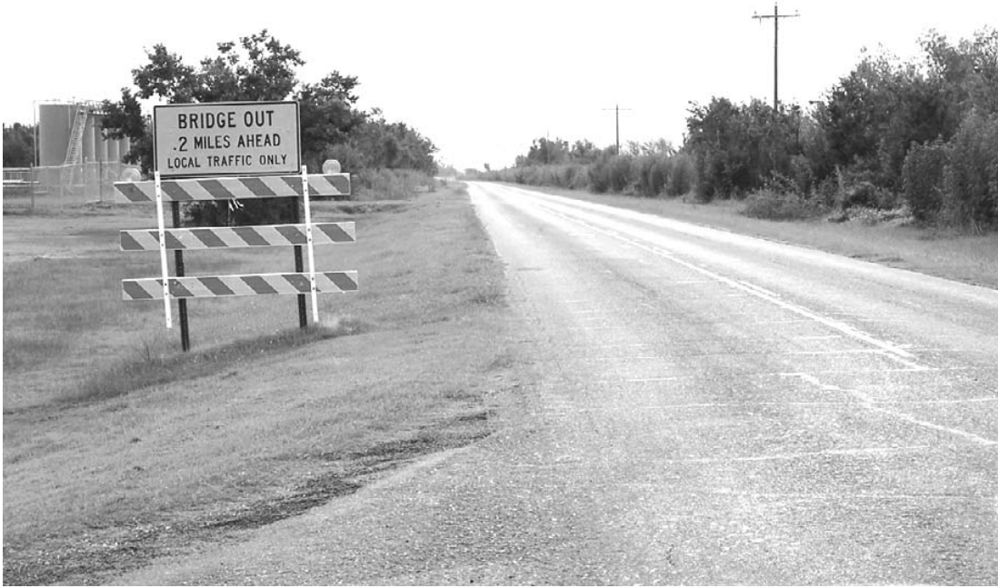
TROSCLAIR ROAD in lower Cameron Parish is slated to be resurfaced and widened to DOTD standards with the aid of $2.4 million in CIAP funds.
