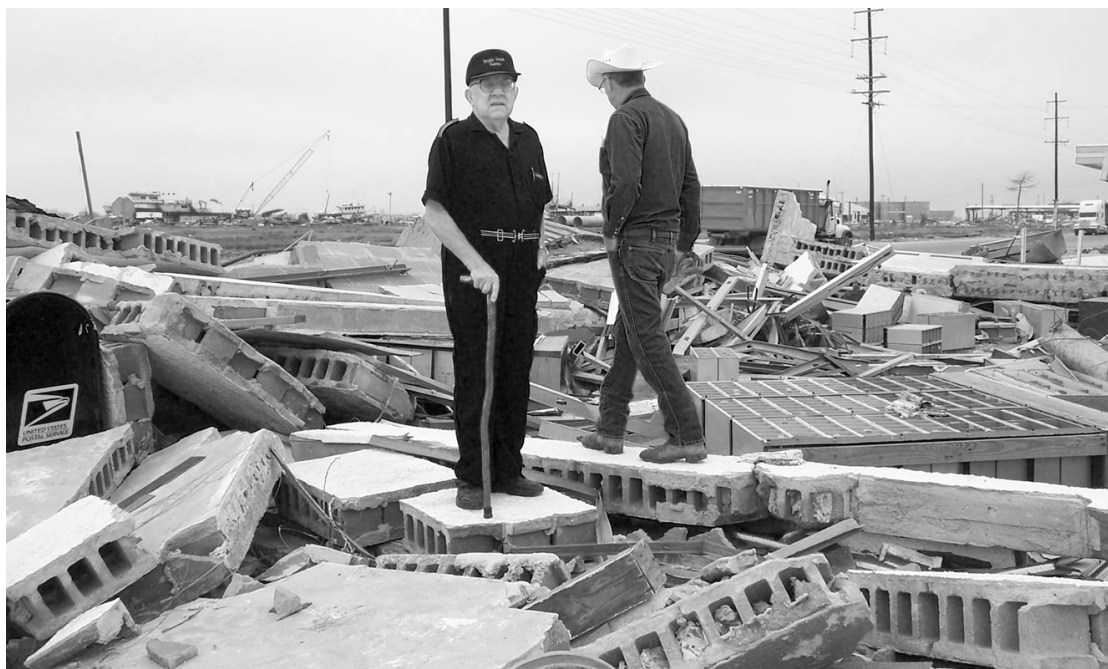
FRANKIE HENRY SURVEYS what is left of the building he had leased to the Cameron Post Office, prior to clean-up. (Photo by Cyndi Sellers.)
