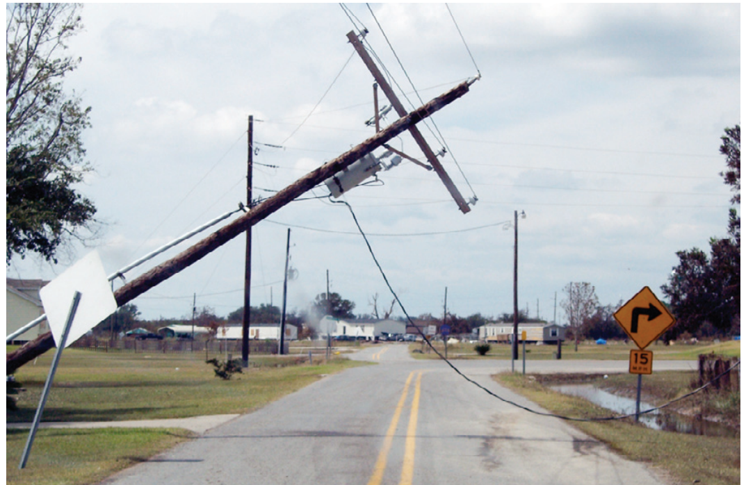
THE DANGEROUS ANGLE of this utility pole creates a hazard for motorists who drive under it. (Photo by Paul Sellers.)
