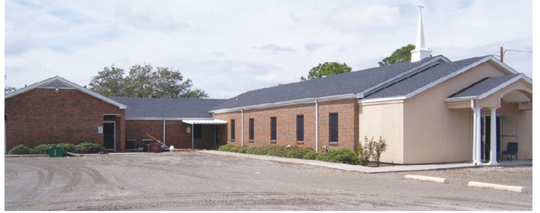
HACKBERRY BAPTIST Church came through the storm in fairly good shape. (Photo by Paul Sellers.)
