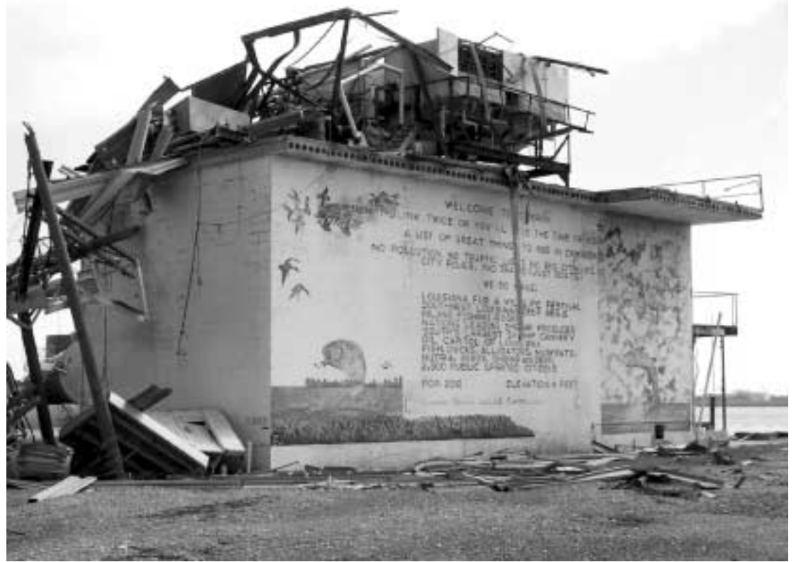
ONE FAMILIAR landmark in Cameron survived the hurricane. The old Bolo Troclair ice plant built of concrete blocks stood up well, as did the mural on its side which was painted some years ago and welcomed visitors to Cameron.
