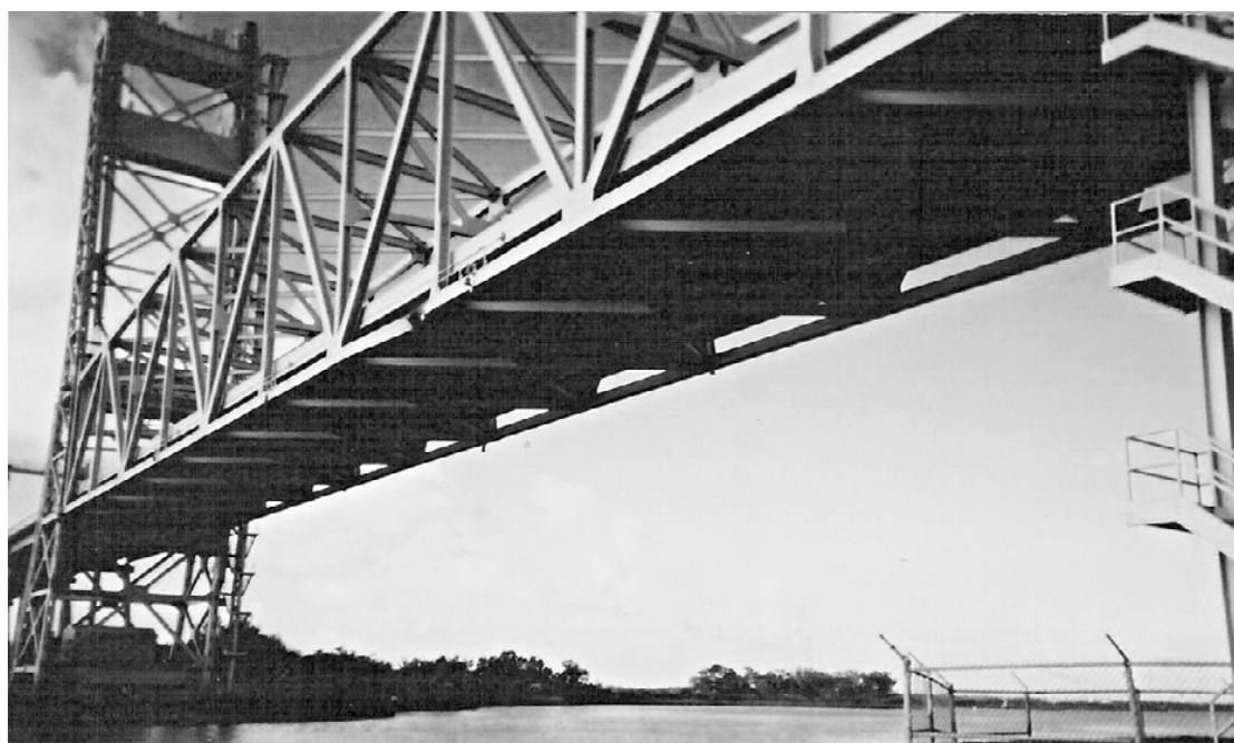
THE ELLENDER BRIDGE just re-opened after being closed due to two barge accidents within a week of each other. Repairs took most of a week before the bridge was re-opened to vehicles.
