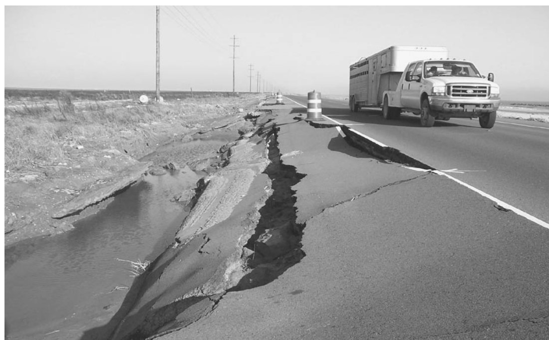
MOTORISTS SHOULD heed the 45 - mph speed limit. Large areas of shoulder damage make driving dangerous. (Photo by Cyndi Sellers.)
